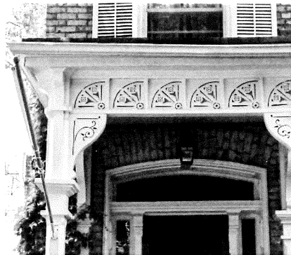
510 Princess Ave. porch detail
