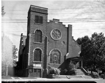
Hyatt Avenue United Church was featured by the Free Press Saturday, June 8, 1946. The building that still stands is empty and deteriorating. Source: London Free Press archives.
