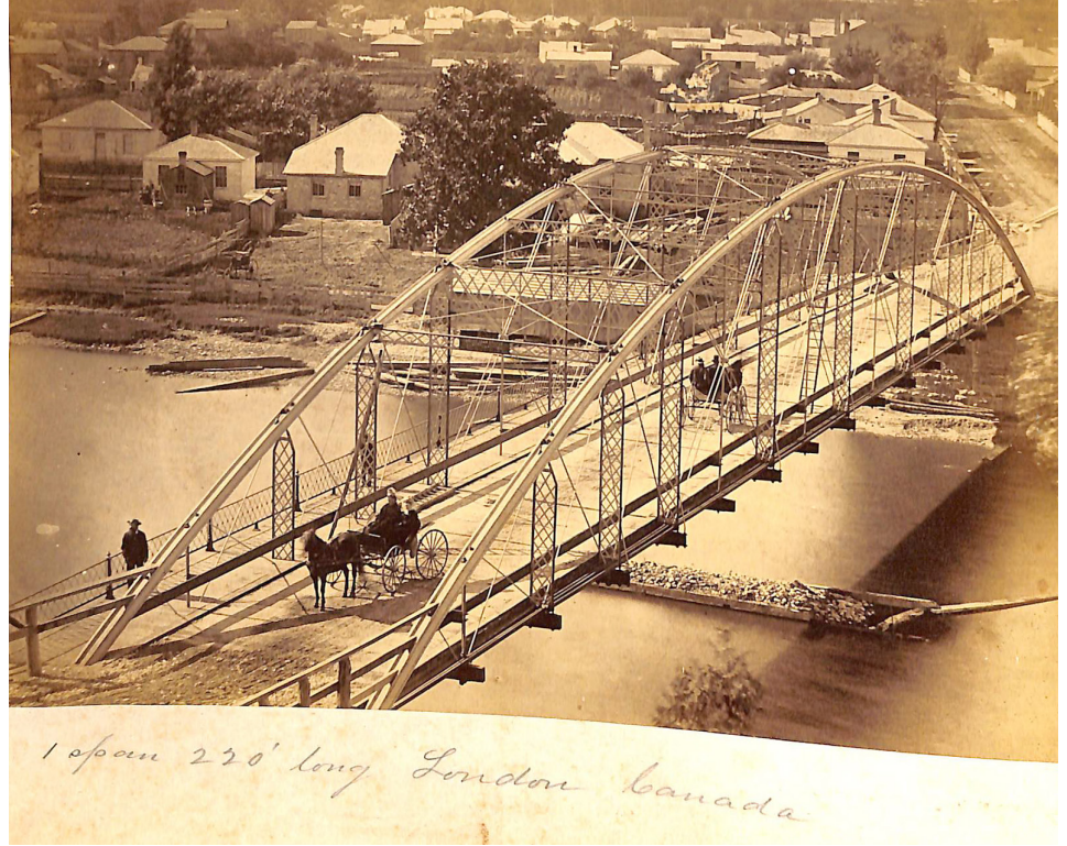
Figure 1. Photograph of Blackfriars Bridge taken shortly after the bridge was erected, with foundations of the centre pier of the previous bridge still visible. (Photograph courtesy of Stanford University Libraries, Department of Special Collections).
