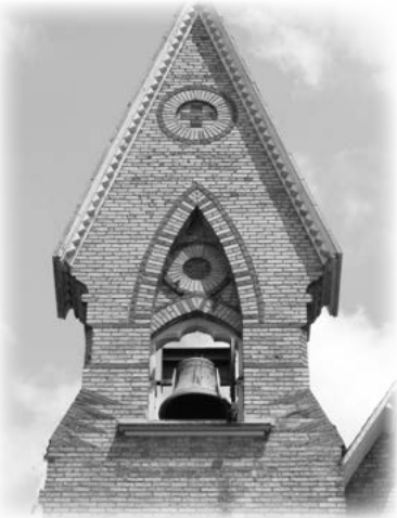
Bell Tower Detail
