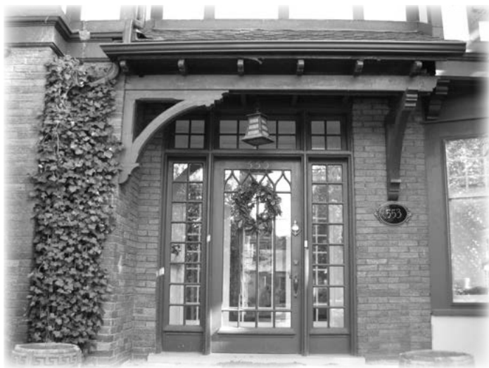
Doorway detail at 553 Dufferin Ave.
