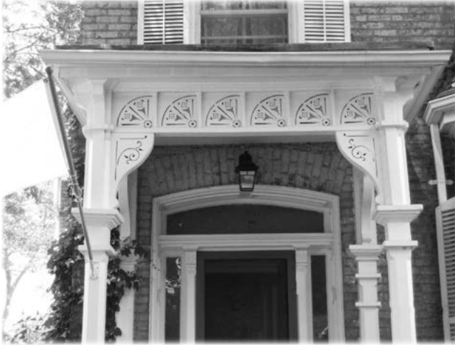
Porch detail 510 Princess Ave.
