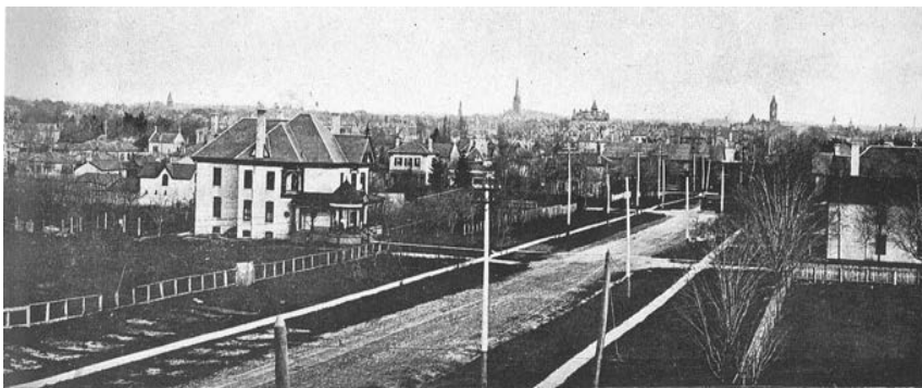
VIEW FROM ST. JAMES STREET, LOOKING SOUTH.
