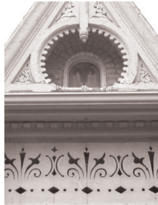
447 Piccadilly St. porch woodwork detail
